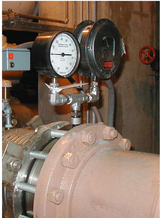
**Dead-band adjustment:** A mechanical Bourdon tube switch with a range of 2 to 60 psi has a minimum dead-band of 3 psi. The solid-state A-B switch with the same range has a minimum Dead-Band of 0.30 psi, a ten-fold improvement in performance.
