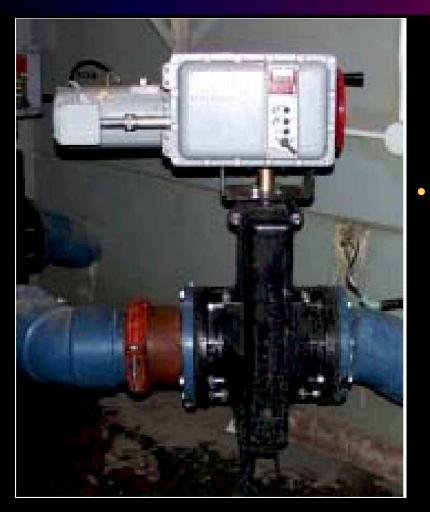
6. The fully enclosed rubber sleeve by the iron body allows the valve to handle high surge pressures.
