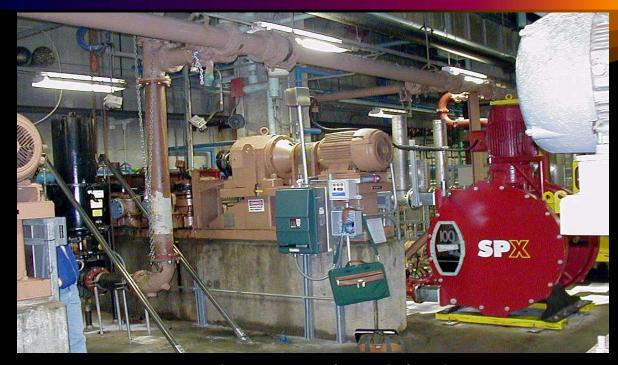
• Watson Marlow Peristaltic hose pump feeds sludge into egg shaped digesters.
