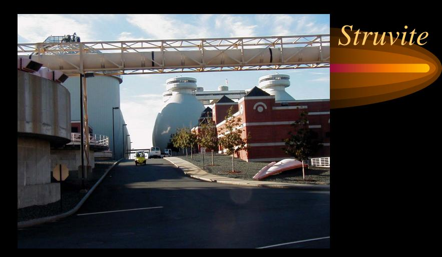
• Boston Harbor WWTP at Deer Island encounters struvite problems on sludge systems. Magnesium originates in the salt air environment.
