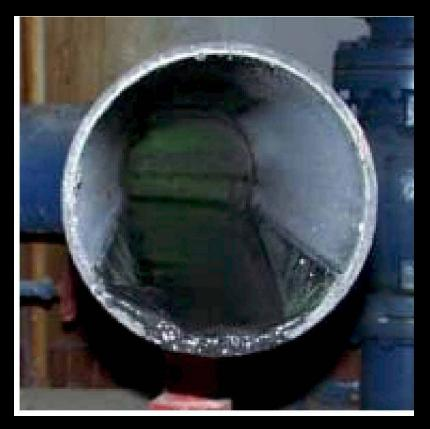
• The piping was replaced with glass lined ductile iron pipe and fittings three years ago, and has proven very successful. The pipe was examined in October and it was observed that there was no struvite buildup inside the piping.
