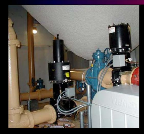
6" DAC with Fail Closed Pneumatic actuator Controlling Raw Activated Sludge and Waste Activated Sludge.
