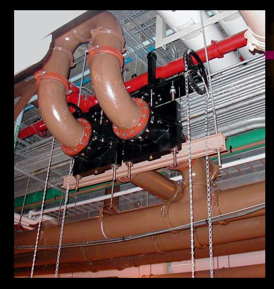
Onyx DHC pinch valves effectively control sludge feed to digesters at 500 ft head pressure.
