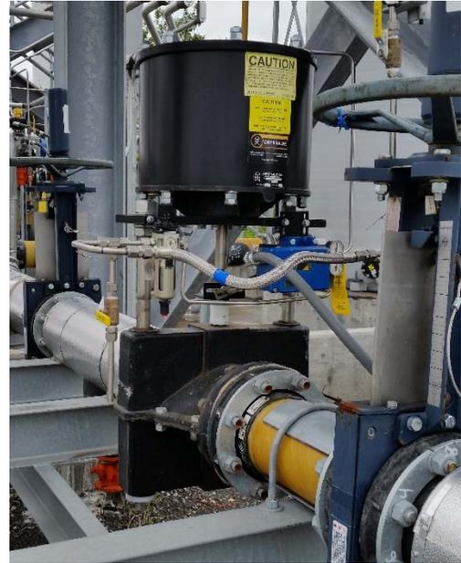
7. Valves for **On/Off** service can be connected directly to adjacent pipe fittings without straight run in or out.
