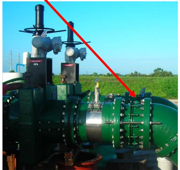
6. On valves **for modulating service**: Allow at least 2-pipe diameters straight run into throttling valves as a minimum.
