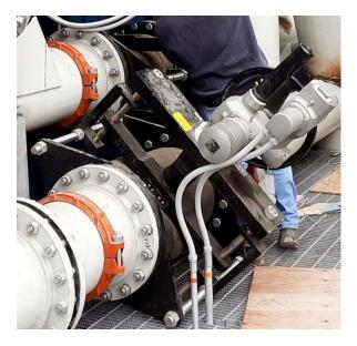
Locate the valve where it can be reached for service and sleeve replacement. Allow access by technicians who may have to calibrate automatic valves. Allow access to the auxiliary hand wheel if valve was so equipped.
