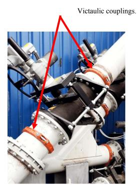
6. On valves for <u>any modulating service</u>: Allow at least <u>2-pipe diameters</u> straight run into throttling valves as a minimum.
