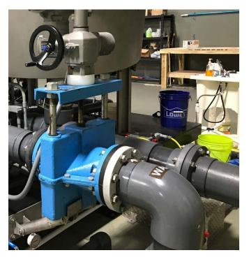
8. Actuator Support for valves installed with horizontal center-line. 2-ways:
