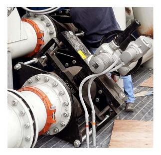
g. Locate the valve where it can be reached for service and sleeve replacement. Allow access by technicians who may have to calibrate automatic valves. Allow access to the auxiliary hand wheel if valve was so equipped.
